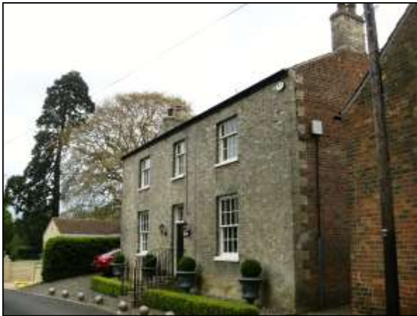
Fig.19 No.6 Spring Lane (Old Solicitor's Place)
